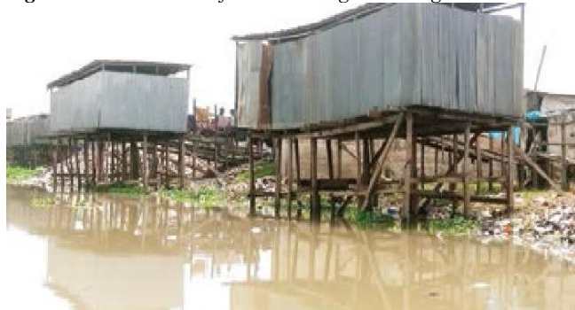
Figure 4: Construction of toilets on Lagoon in Lagos State
